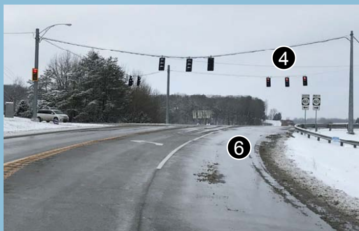
US 150 (looking west)
